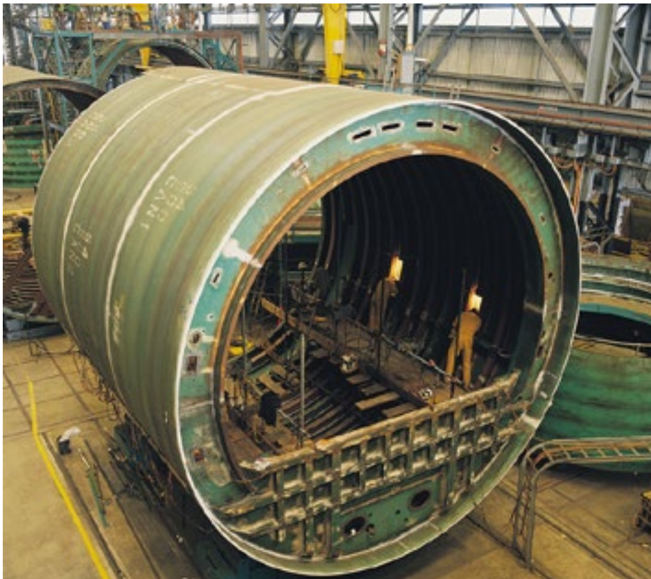
This photo shows the production of 'cans' (individual elements of pressure hull, lying on their side in right background) being assembled into a pressure hull section with 3 'cans'. Image courtesy of ASC Pty Ltd.
